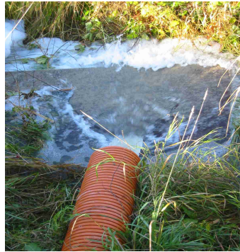
Clear return water from the 3rd sedimentation pond flows back to the lake
