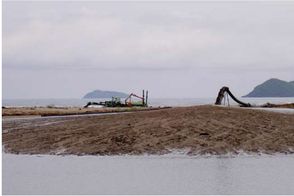
The Watermaster carrying out a maintenance dredging operation.
