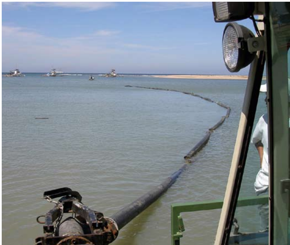
The Watermaster performing suction dredging in the river mouth.
