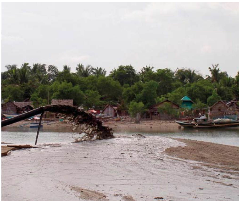
End of the discharge pipe.
